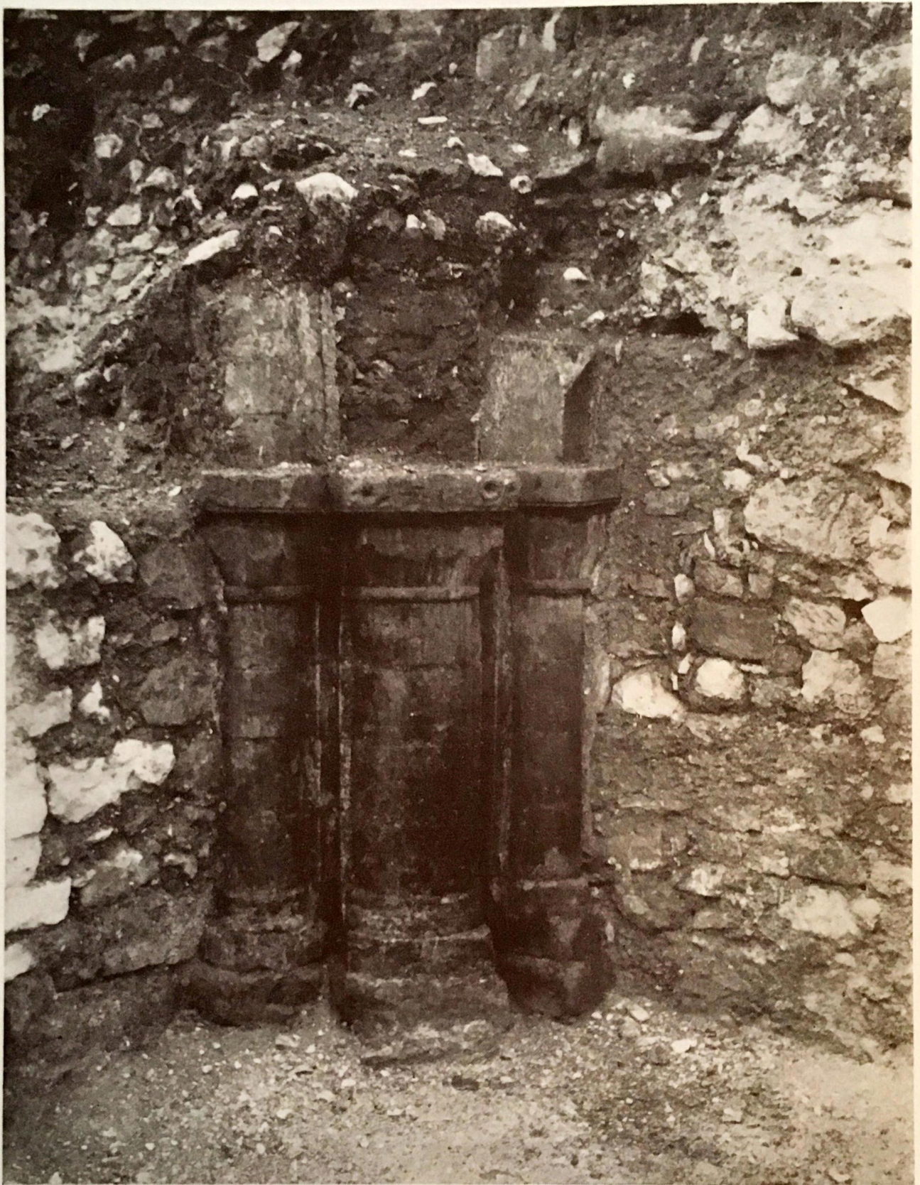
UNDERCROFT OF CELLARERS' LODGING : GROUP OF TRIPLE STONE SHAFTS
